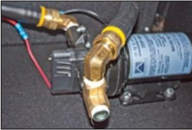
**Feature:** 5.0 GPM, 12-volt, 1.9 AMPS, 60 PSI diaphragm feed pump with a pressure switch tucked under a removable panel located in the locked, steel control panel and storage area.
